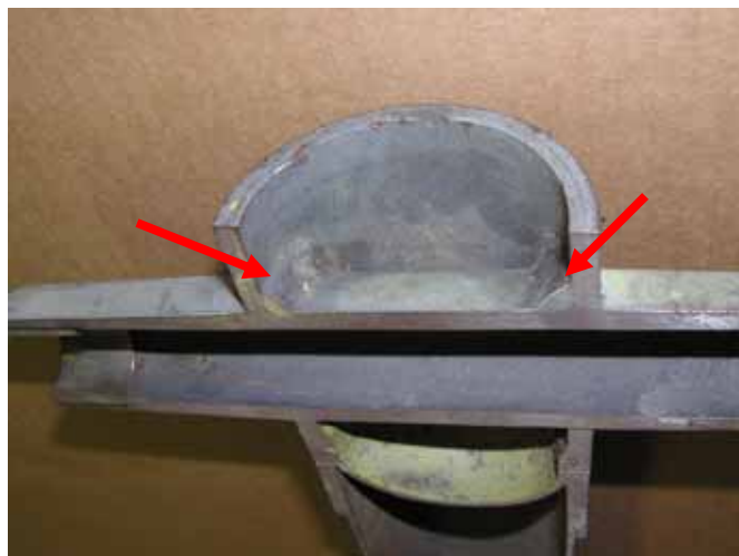
Fig. 7 Magnetic particle inspect for cracks and separation.
